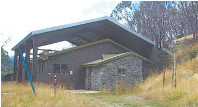
'Old' Tiobunga characterised by its second roof before a total rebuild commenced in 2007 (photo by Department of Planning).
