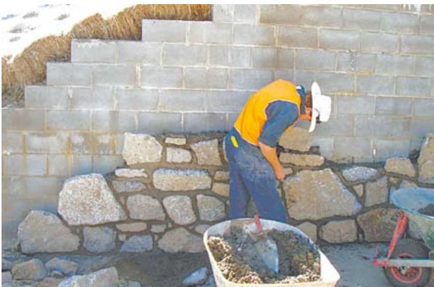
Stonemason at work on the toilet entry (photo by Tim Greville).
