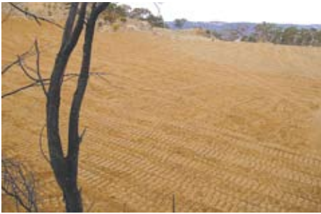
Final capping layer in late 2004 prior to planting (photo by Dave Woods).
