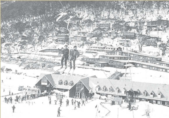
Thredbo Village and front slopes in 1964 (source: Exploring EarlyThredbo).
